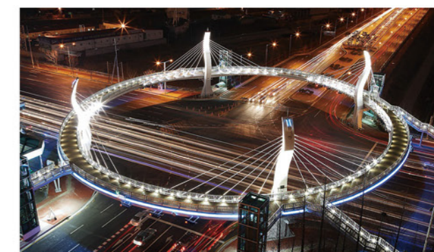
韩国·水原·过街天桥 KOREA, SUWON OVERPASS
